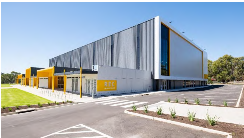
Reynella East College Redevelopment - New Gymnasium
