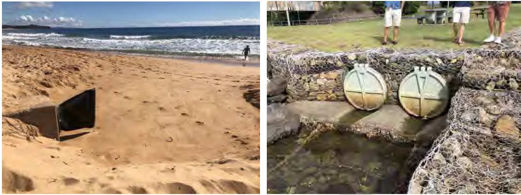
Figure 5-6 Left: Example of a duckbill outlet treatment at Collaroy Beach, NSW. Right: Example of one-way tidal flaps at an estuarine stormwater outlet in Coffs Harbour, NSW
