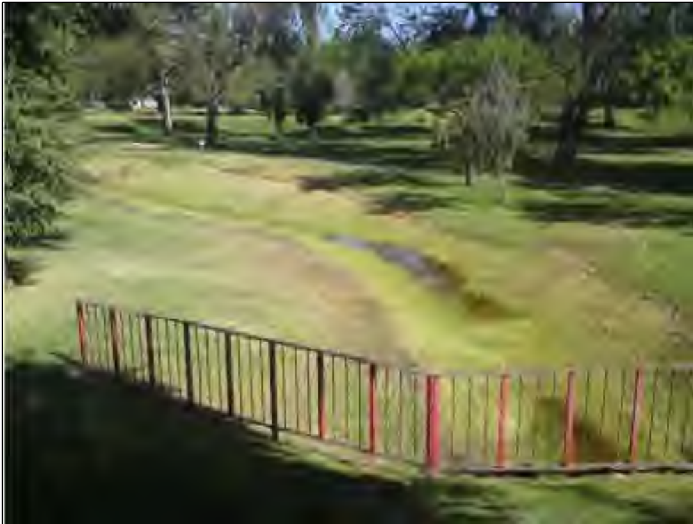
Figure 5-4 Grass swale in Rymill Park – (Source: Chapter 11 - Swale and Buffer Strips, Water Sensitive Urban Design Technical Manual Greater Adelaide Region)
