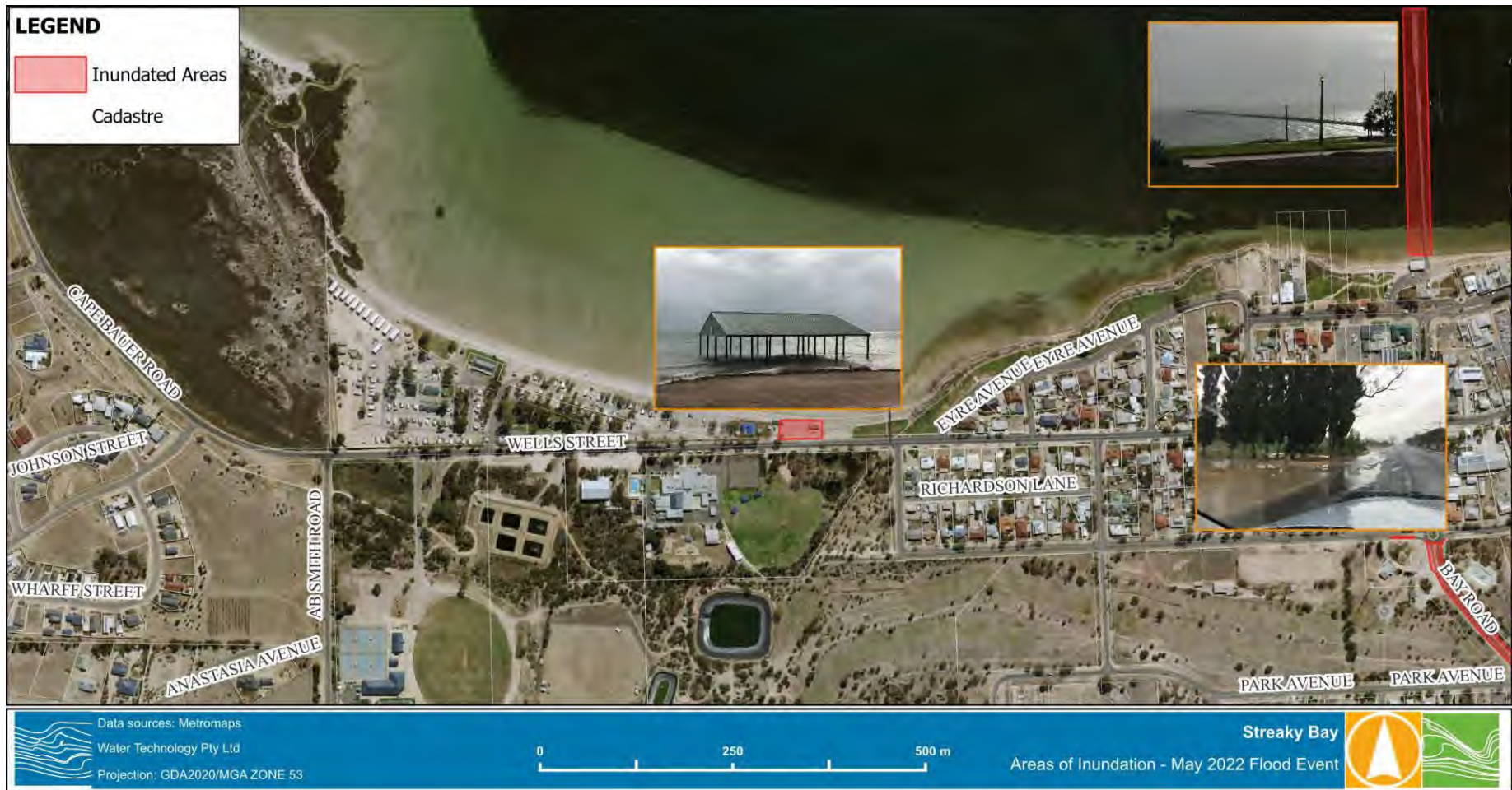
Figure 4-9 Inundated Areas around Wells Street – May 2022 Flood Event
