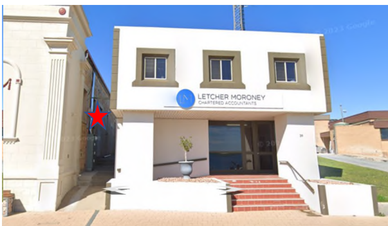
View from Front of Hall to Hall Meter Box Location (Alfred Terrace)
