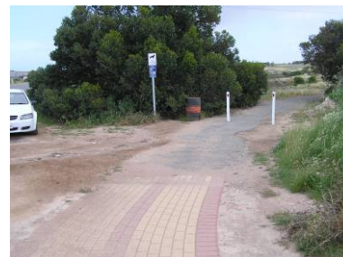
Southern end of shared path. Note the lack of information/directional/distance signage.
